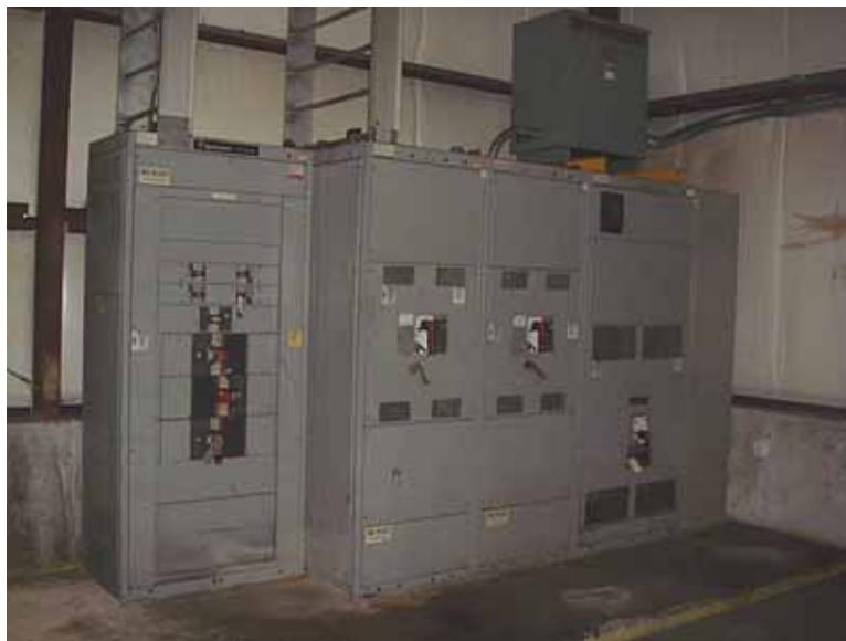
One of three high voltage power regulators for former production area
