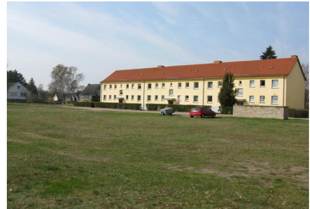
Open area between the buildings
