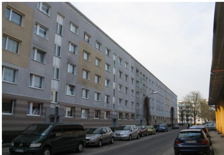
Front side of the building
