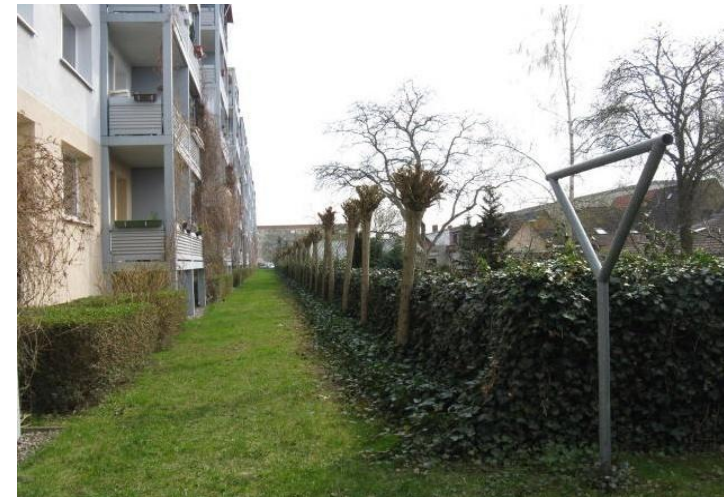
Rear side of the building
