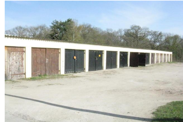
Parking garages on the site
