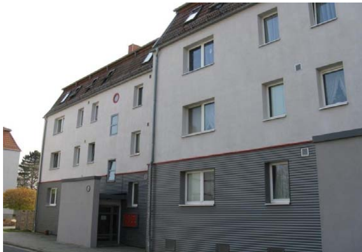
Rear of the building
