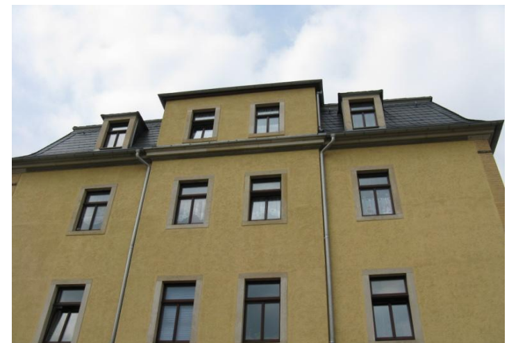
Rear of the building
