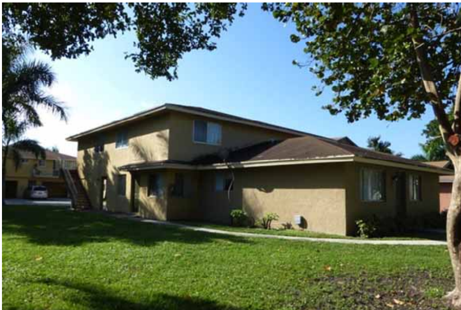
Typical fourplex within the Delray Estates condominium
