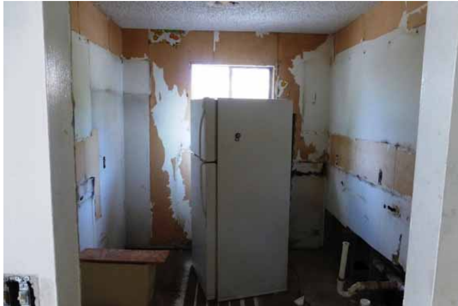
Uninhabitable unit under renovation
