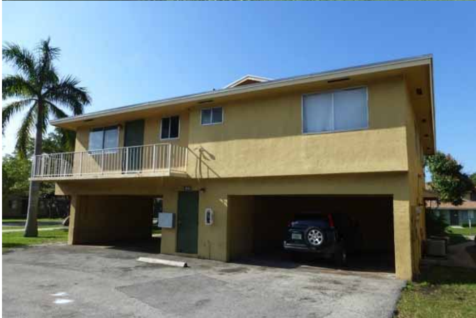
Typical fourplex within the Delray Estates condominium
