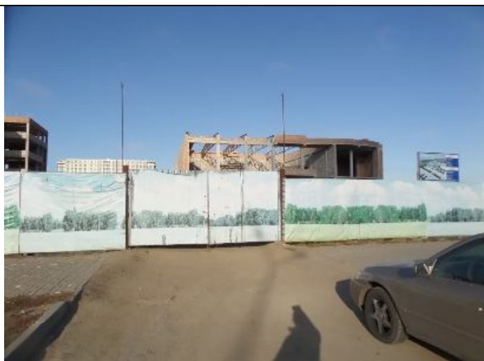
Construction of the restaurant
