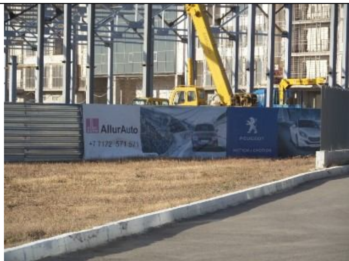
Construction of the autocenter
