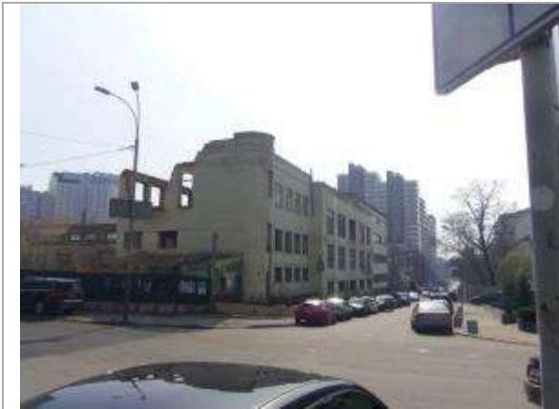
View on the site from A. Barbyusa and Tverska Streets intersection (south-western part)
