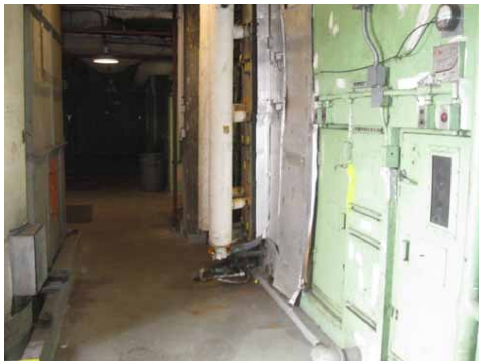
TYPICAL ROOF MECHANICALS
