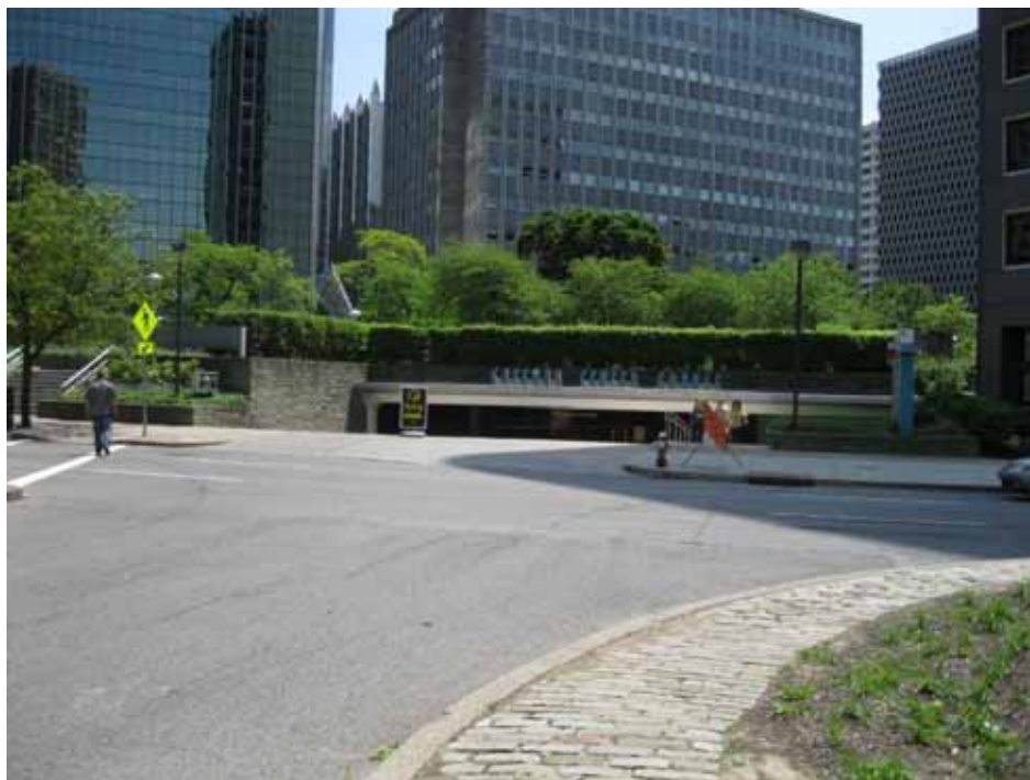
PARKING GARAGE ENTRANCE
