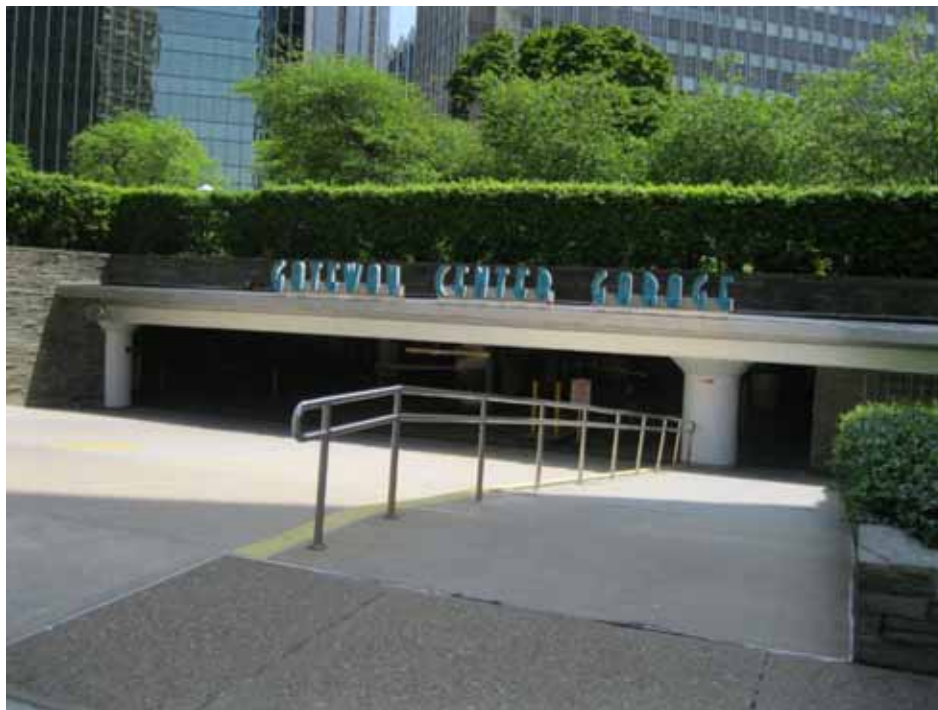
PARKING GARAGE ENTRANCE
