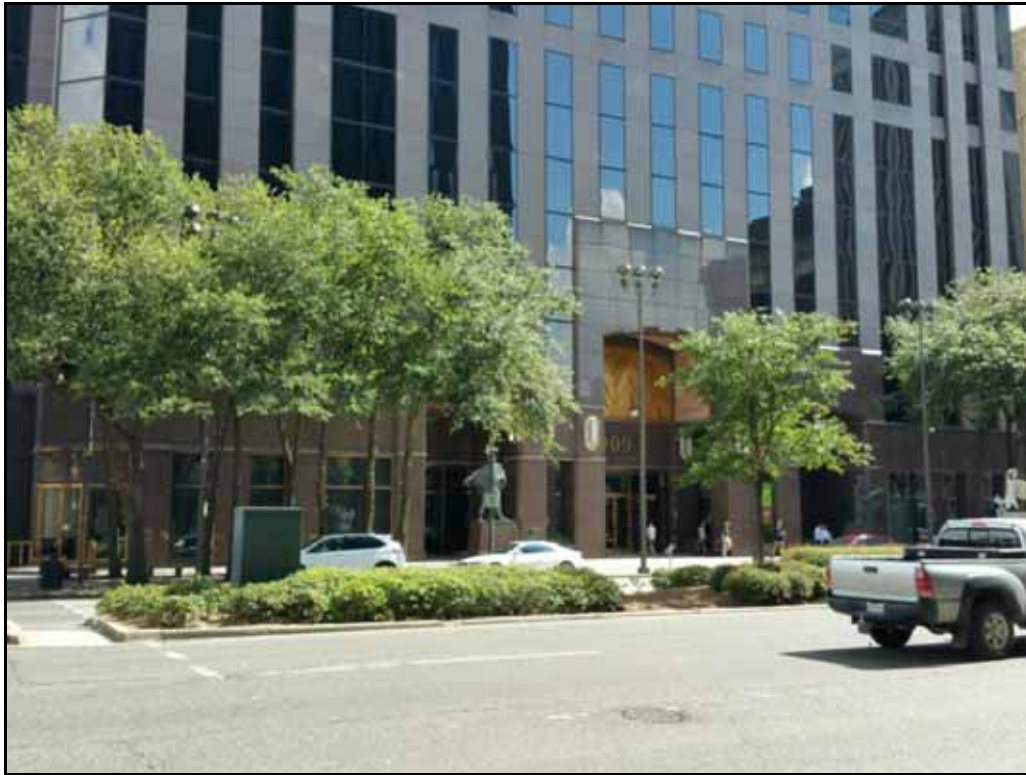
Figure 8: Typical Exterior View
