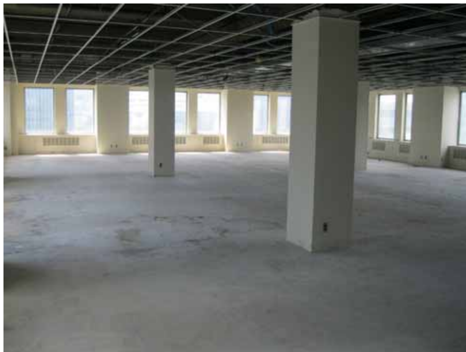
TYPICAL OFFICE SPACE – UNFINISHED
