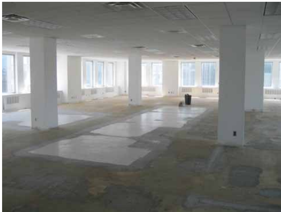
TYPICAL OFFICE SPACE – UNFINISHED
