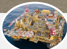
FPF-1 Production Facility
