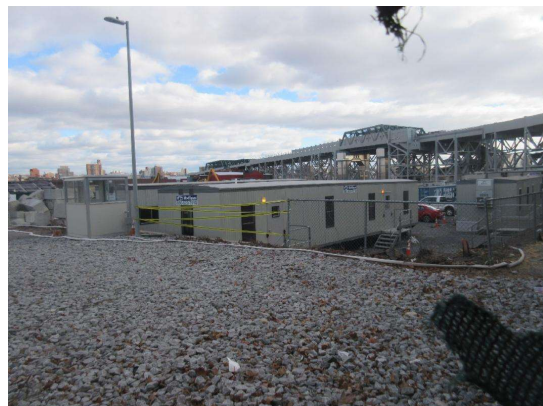
Inside View of the Property
