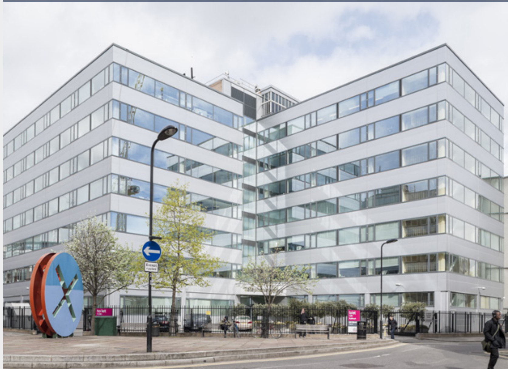
Shoreditch - TELEPHONE HOUSE
