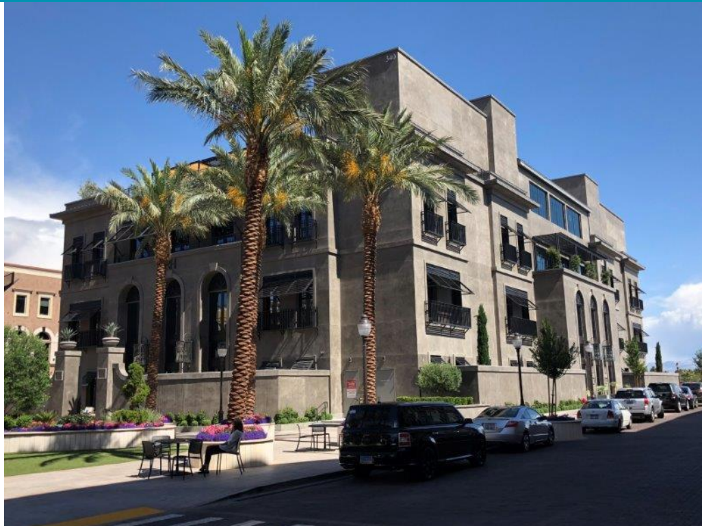
VIEW LOOKING NORTHWEST AT RESTORATION HARDWARE
