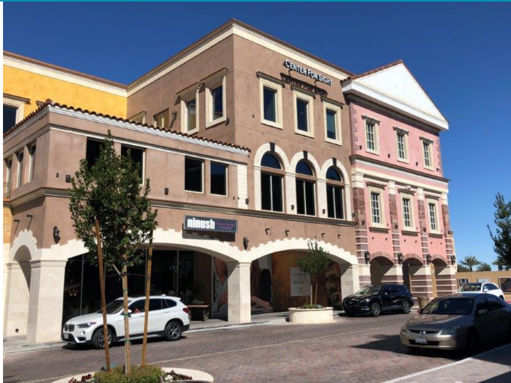
VIEW OF TRIAD B IMPROVEMENTS
