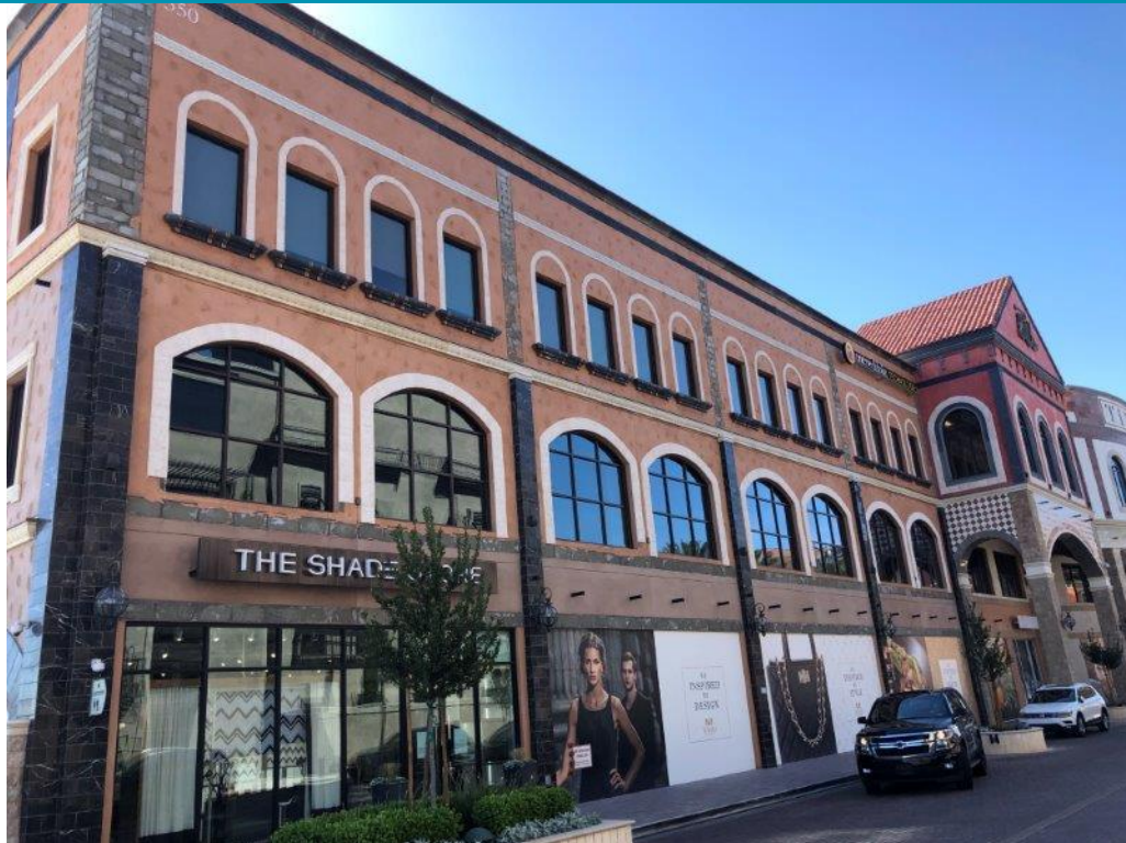
VIEW OF TRIAD B IMPROVEMENTS
