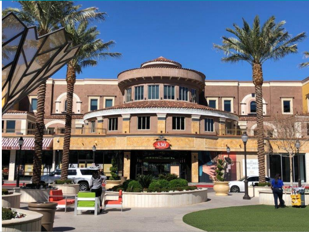
VIEW OF TRIAD B IMPROVEMENTS
