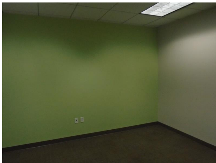
INTERIOR OFFICE AREA
