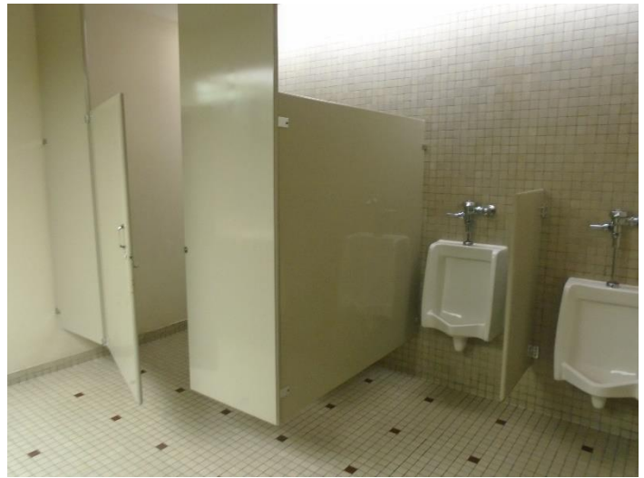
INTERIOR RESTROOM AREA
