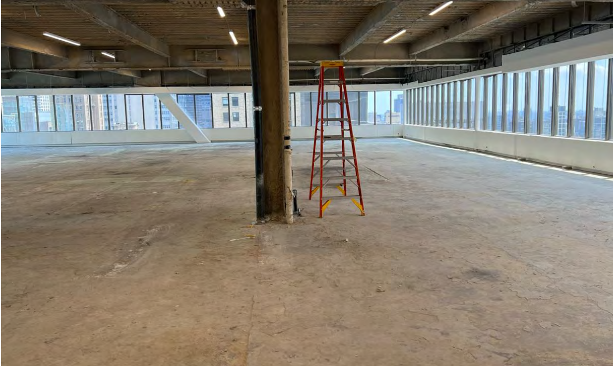
View of the Subject Vacant Office Space
