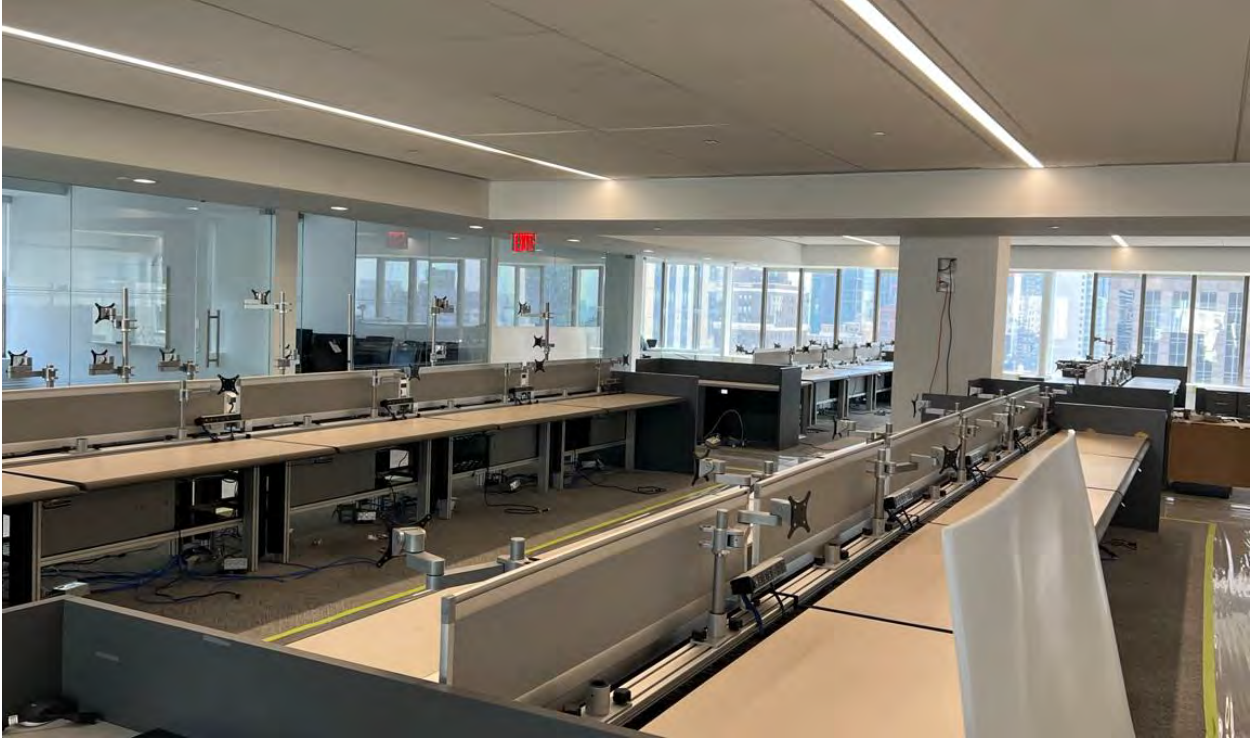
View of the Subject Office Space (Under Construction)
