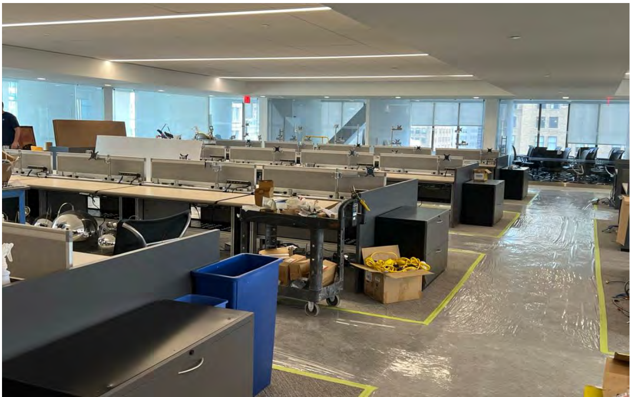
View of the Subject Office Space (Under Construction)
