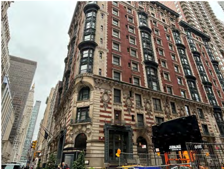
Exterior (Front) - West 28th Street/Madison Avenue
