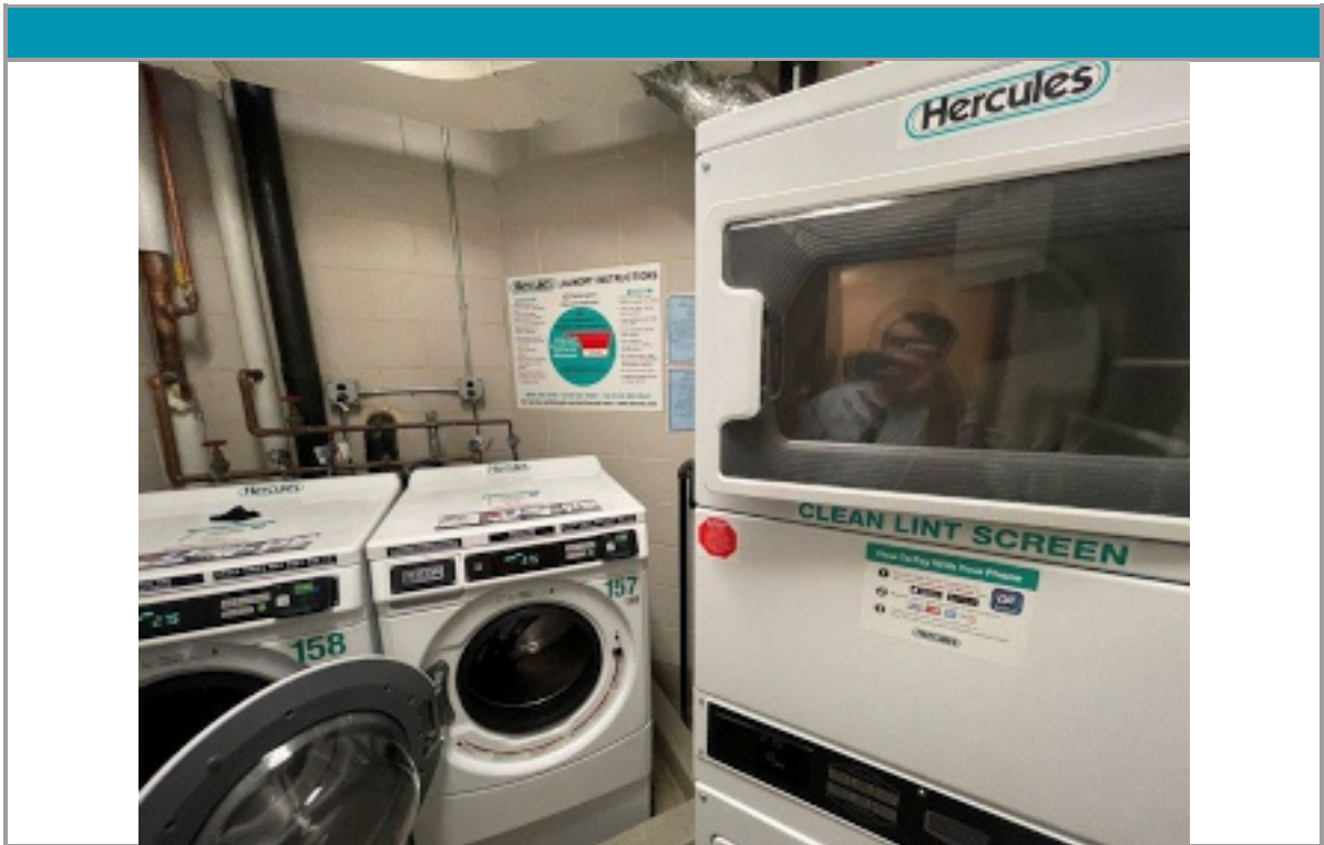
View of a common laundry room
