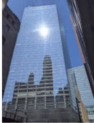
Building exterior (Photo Taken on June 18, 2024)
