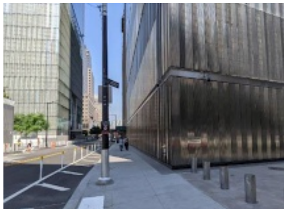
Building side along Vesey Street (Photo Taken on June 18, 2024)
