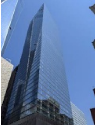
Building Exterior (Photo Taken on June 18, 2024)
