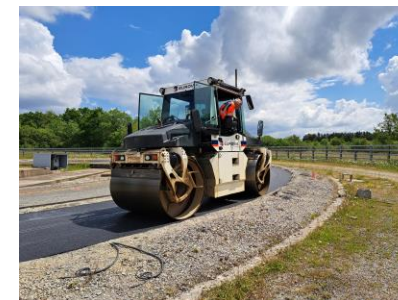
Asphalt and compaction
