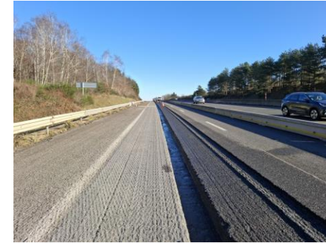
Road milling & trenches
