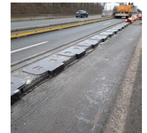
Coils laying & gluing
