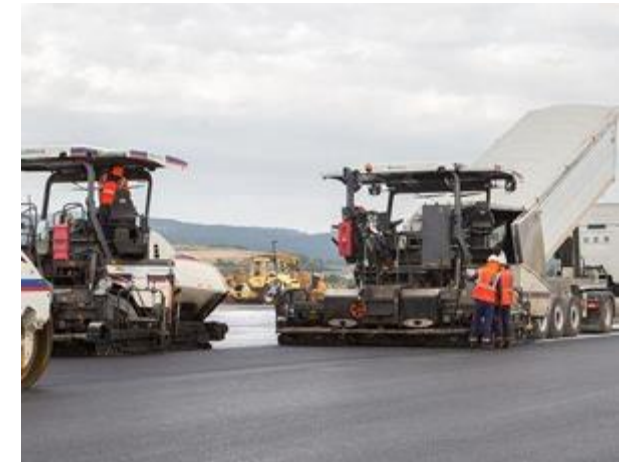
200m surface course repair test
