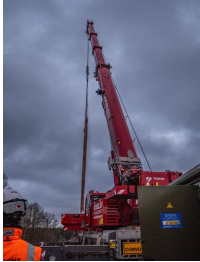
Installation of electric station
