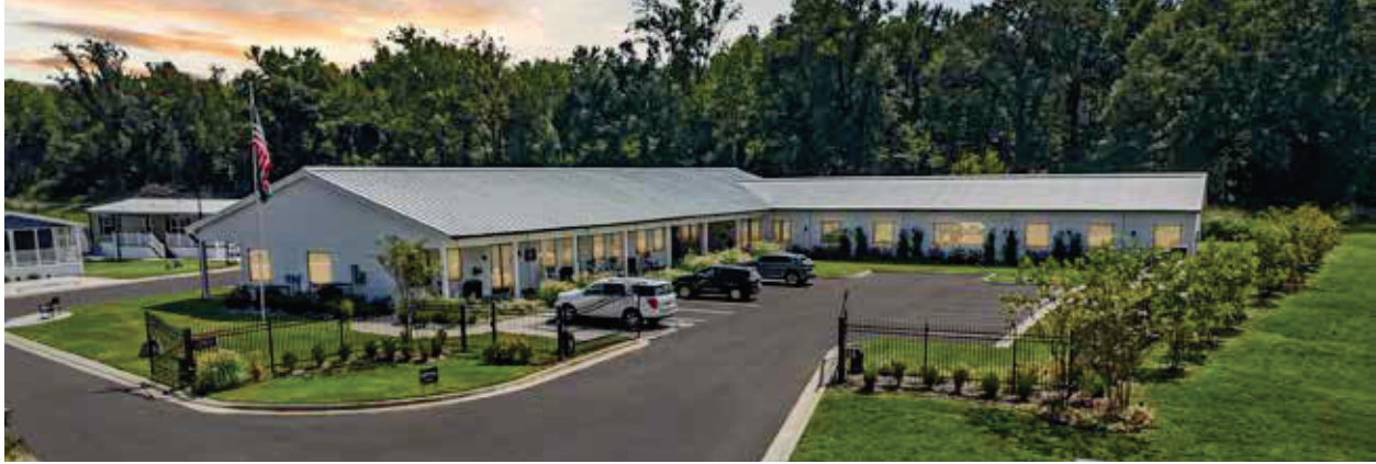
RIVER BLUFF ESTATES & OFFICE OF UMH SALES AND FINANCE, INC., Memphis, TN Developed in 2024
