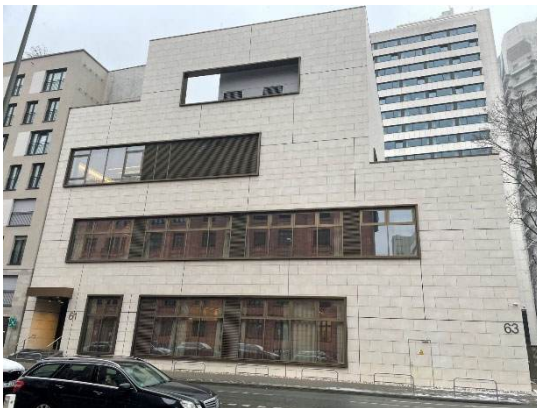
Building extension/rear elevation (2025)
