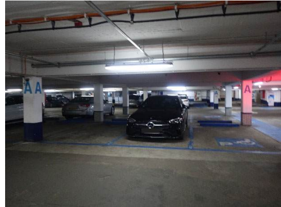
Underground car park (2024) (not subject to valuation)
