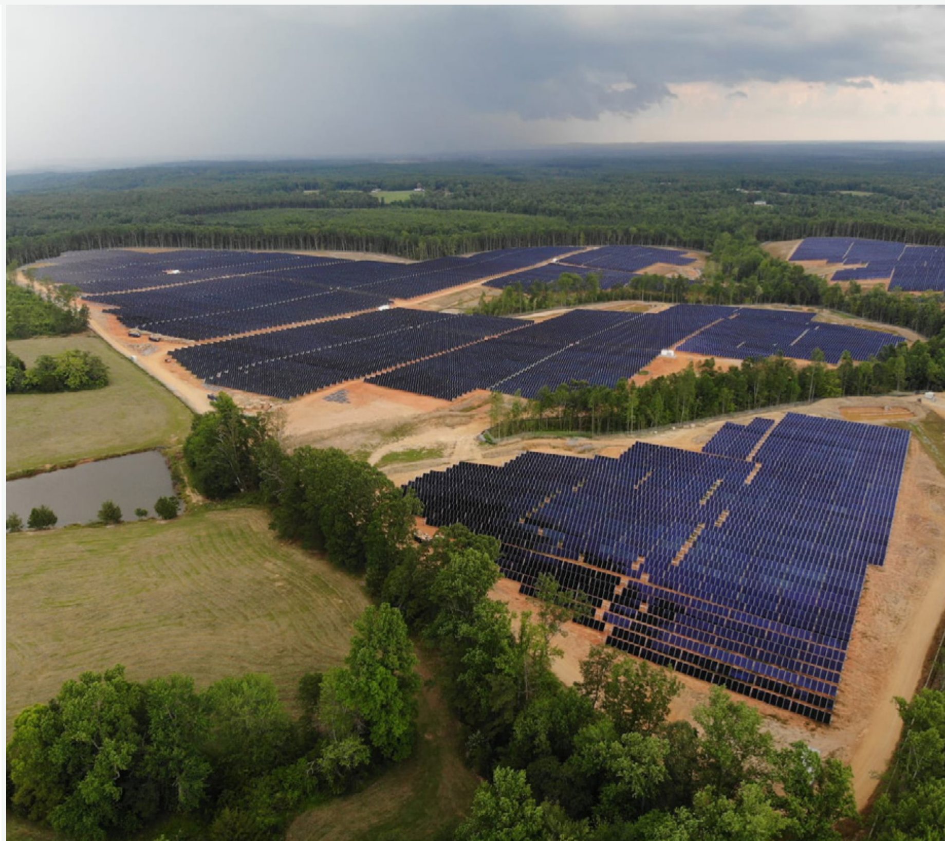
Energix / Pamplin / Virginia, USA
