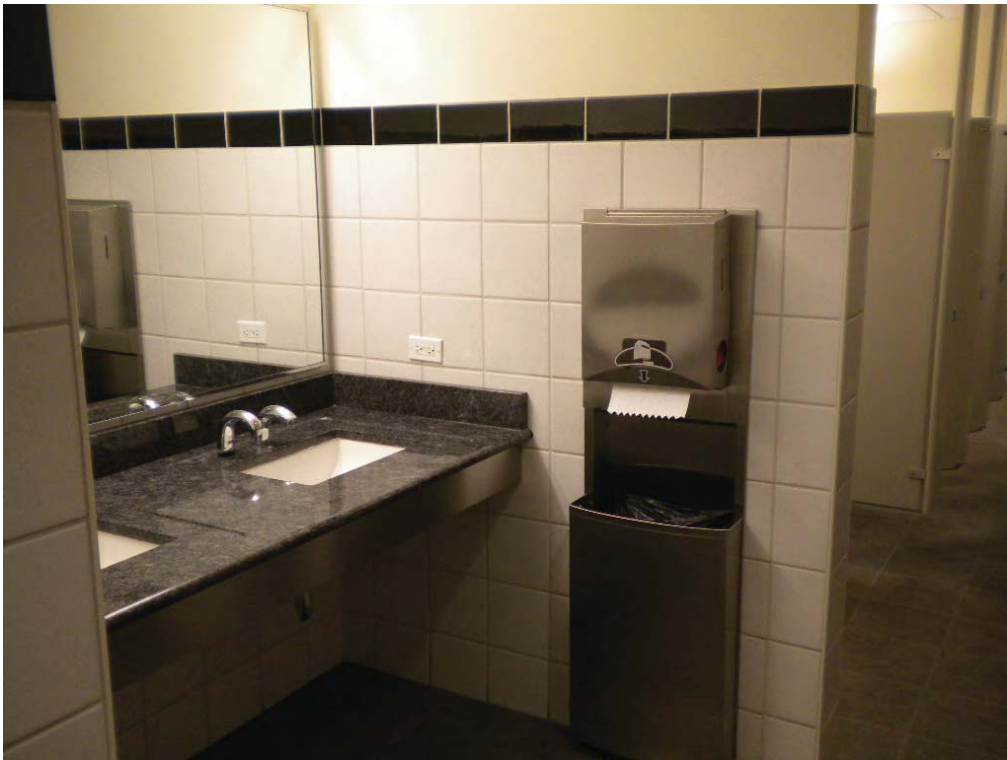
VIEW OF A TYPICAL RESTROOM FACILITY
