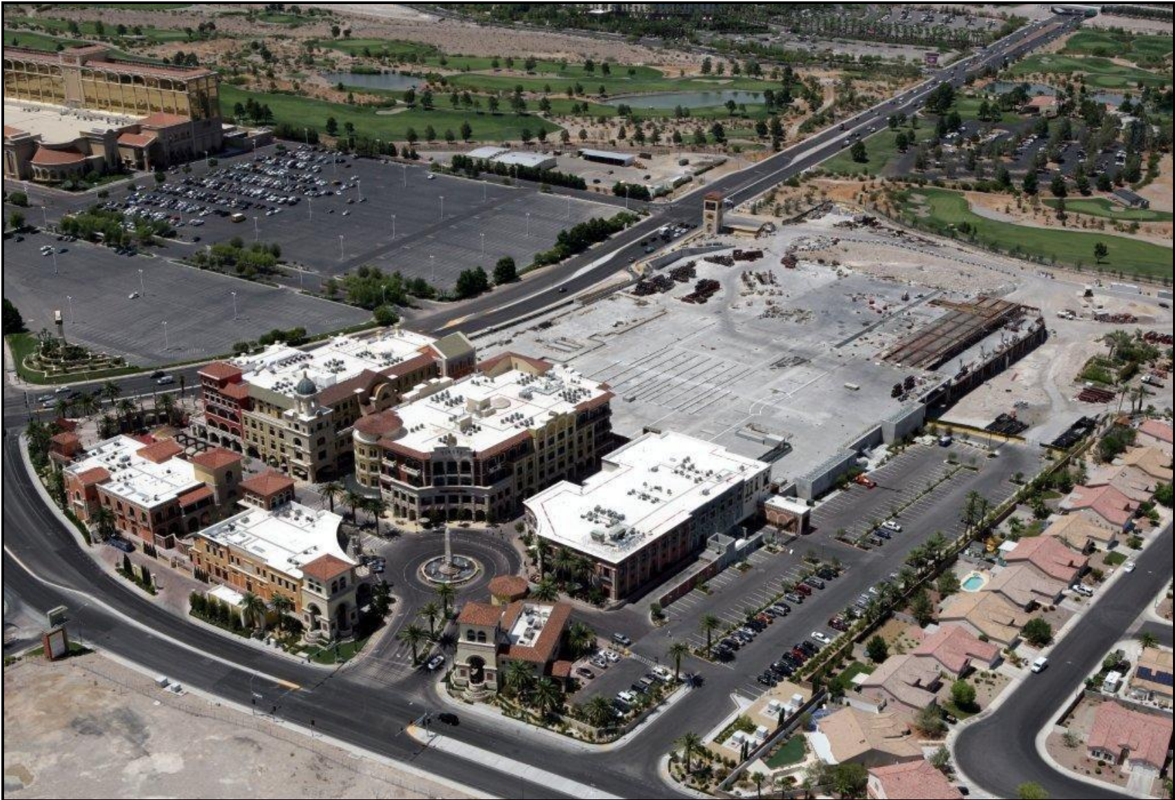
Aerial View of Current Improvements & Ongoing Construction of Tivoli Village
