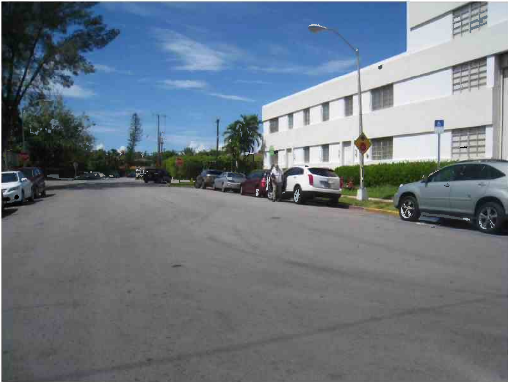
SOUTHERLY VIEW OF SHERIDAN STREET
