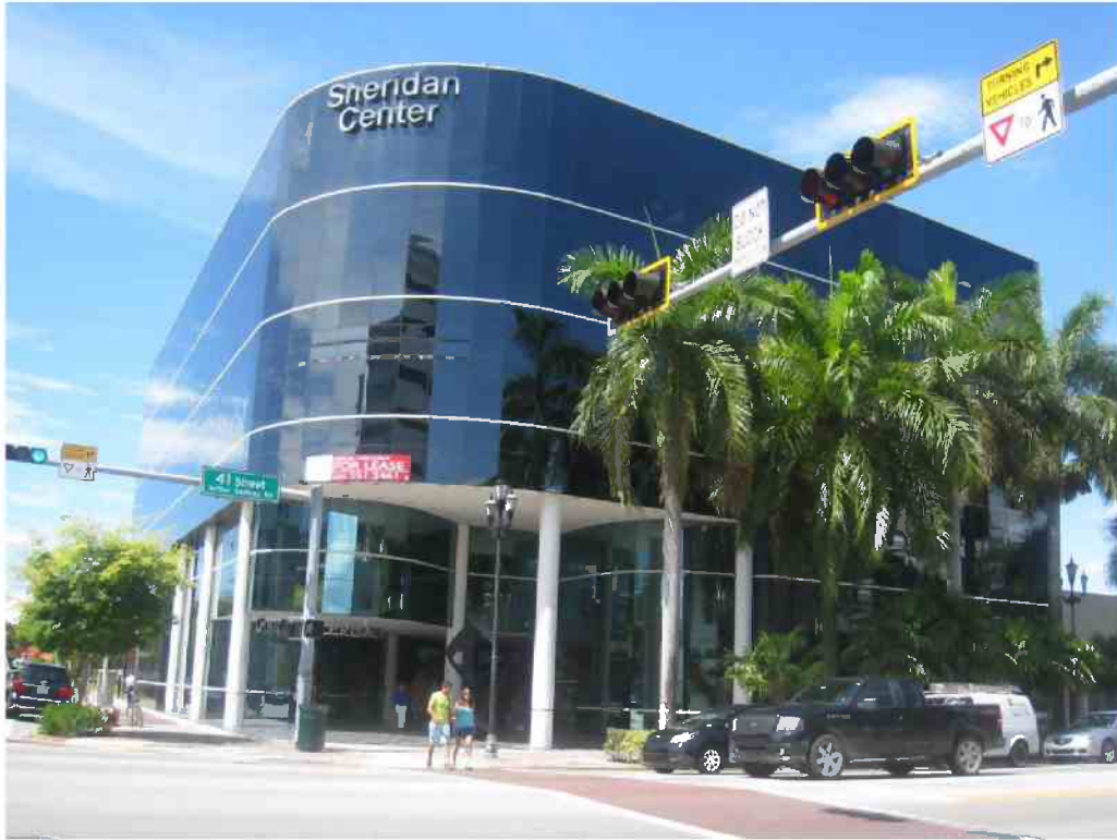
FRONT OF SUBJECT PROPERTY
