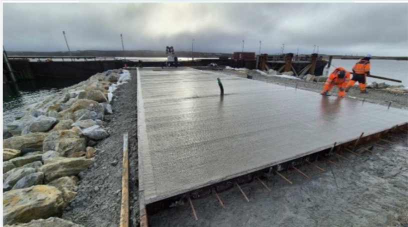
Completion of the concrete surface on the pier access road
