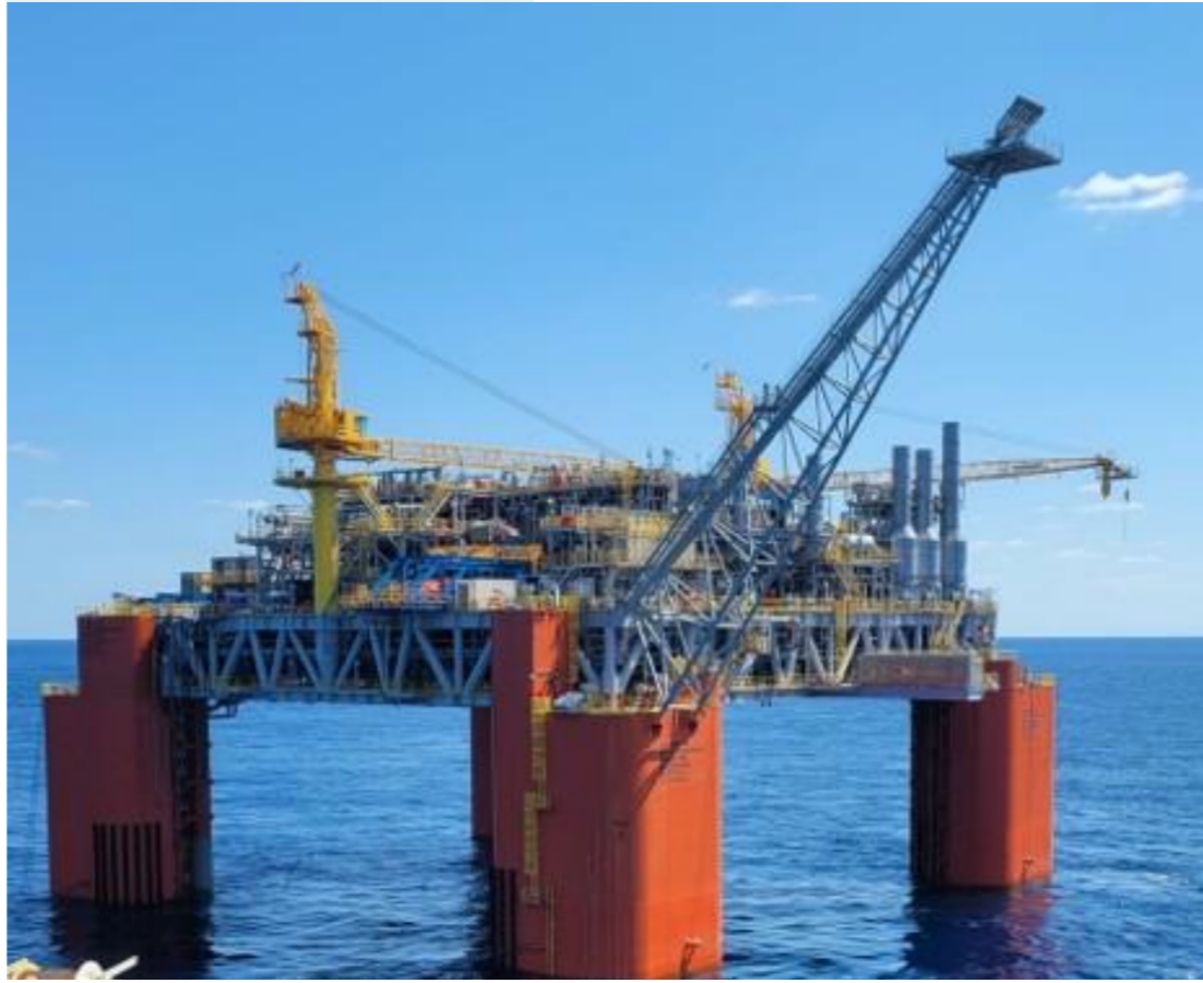
Floating Production System Treatment and Production Facility - Shenandoah Hub
