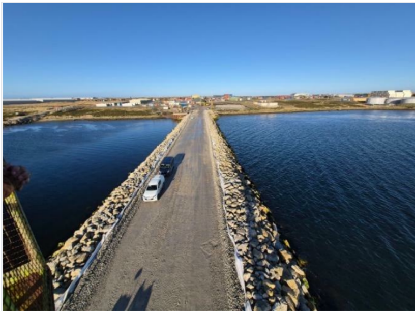
Completion of the stone battery on the pier access road
